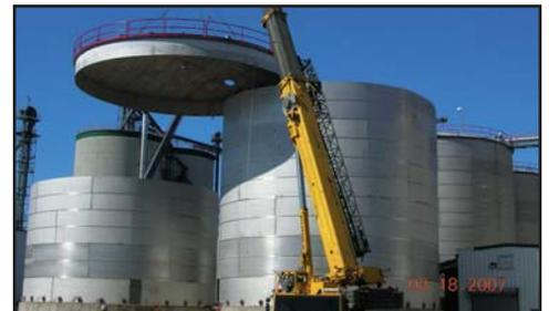
Wimbc0, Inc. installs the lid for one the additional fermentors needed for plant expansion at GLE.
