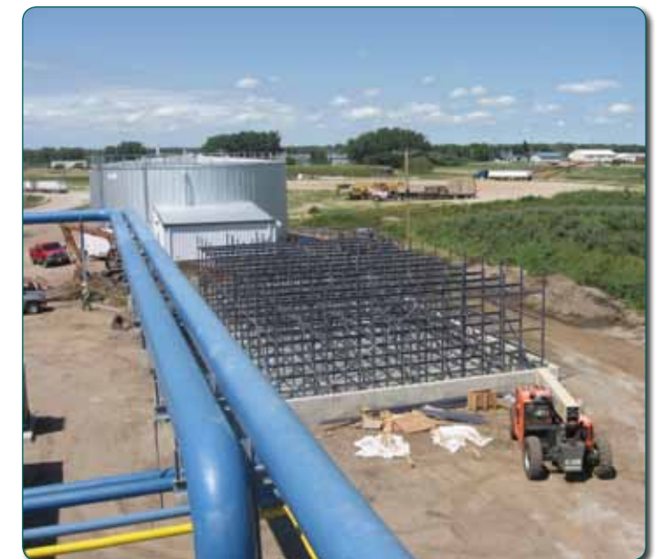
The Watertown cooling tower under construction.
