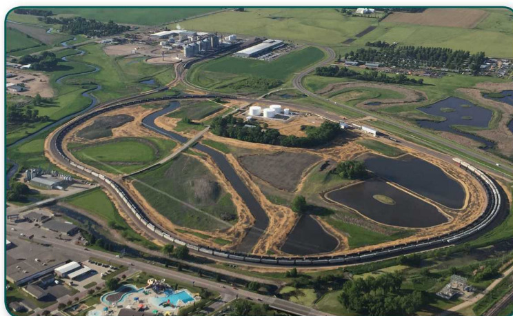
Watertown and Mina can reach export markets via shipping a unit train of ethanol. Pictured here is the Watertown loop track completed in 2016.
